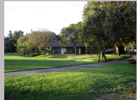
Integrated with the above-ground drainage system, the community center sits at the edge of the largest park in Village Homes
